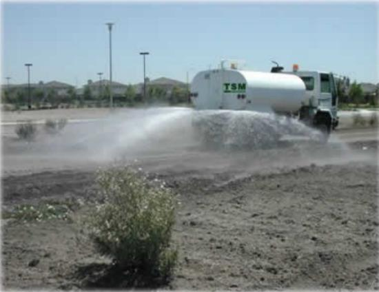
**Sprinkling:** Apply so that the soil is wet but not saturated or muddy and so that air quality requirements are maintained.
