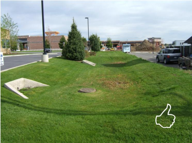
Specifications for swale construction should state the earliest point in construction progress when storm drainage may be directed to the swales, and the means by which this delay in use should be accomplished. Due to the wide variety of conditions encountered among projects, each should be separately evaluated in order to postpone use as long as reasonably possible. (Shallow injection wells must be registered with PHD)
