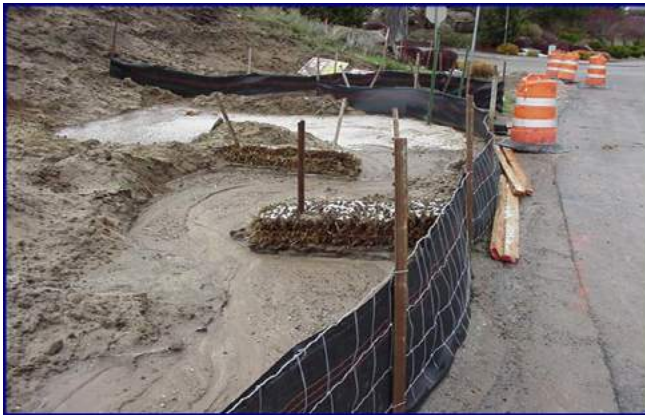
Figure 6-13. A situation where erosion prevention was inadequate, resulting in this silt fence trying to hold back too much weight. This fence blew out moments after the picture was taken.
