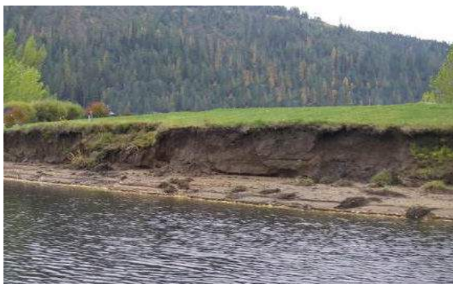
Figure 10-6 Bank erosion caused by boat wakes and flooding. Bank lacks a healthy vegetative buffer.
