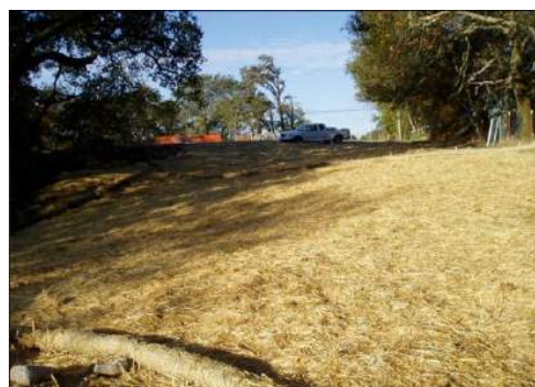
Figure 6-8. Bare soil mulched with straw.
