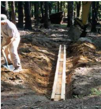
Figure 7-8. Open-top box installation.
