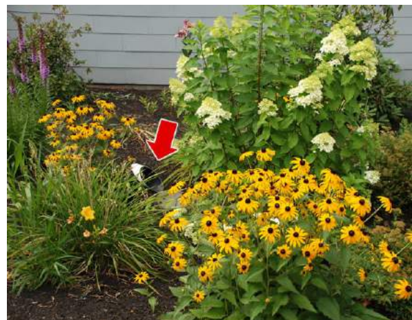
Figure 1-6. A rain garden installed below a downspout.
