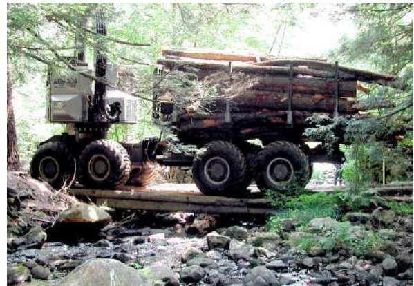
Figure 8-9. Temporary stream crossing.
