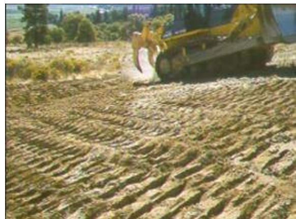
Figure 6-12. Slope roughening with grooves perpendicular to the slope.
