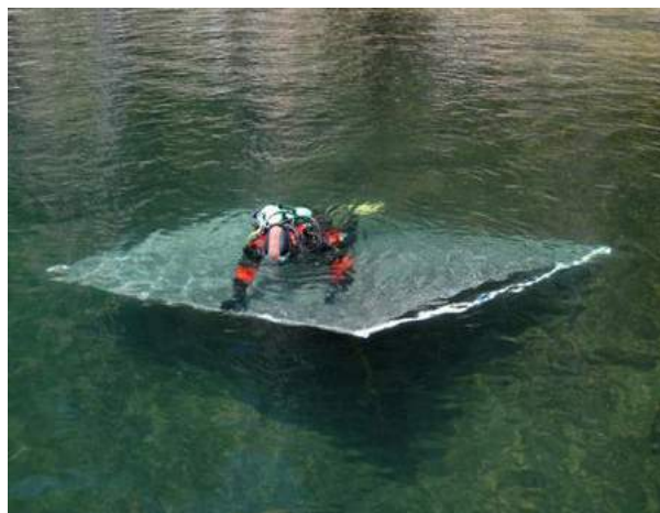
Figure 9-8. Diver installing a 10' x 10' bottom barrier.
