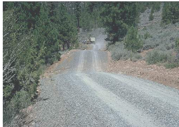
Figure 7-6. Road constructed with outward sloping rolling ditches.
