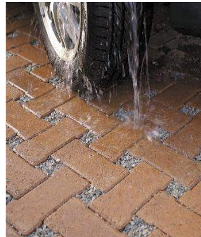
Figure 1-9. Permeable pavers on driveway allow stormwater to infiltrate.
