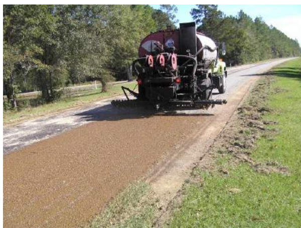
Application of liquid calcium chloride.
