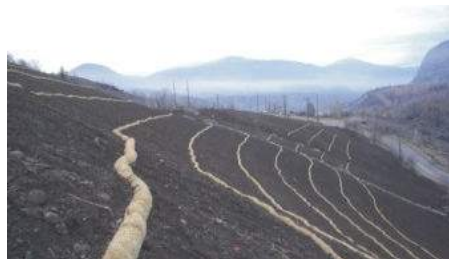
Figure 6-15. Fiber rolls installed perpendicular to flow.
