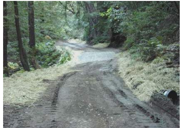
Figure 7-5. Exposed soil has been mulched.
