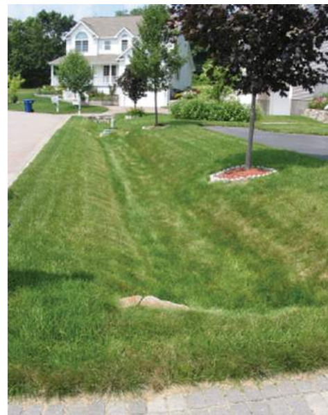
A grassy swale in a residential neighborhood treats runoff from driveways, roads, and roofs.
