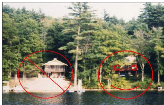
Figure 2-3. The property on the left leaves sloping bare soil/sand exposed to stormwater . The property on the right is attractive with abundant plants and access.
