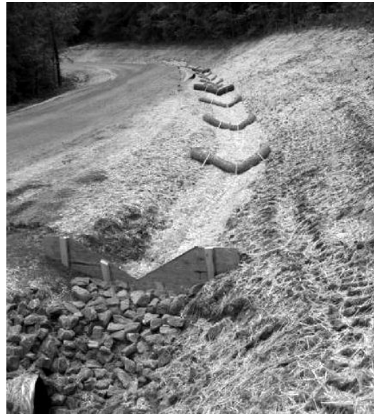
Figure 7-17. Straw/fiber wattles used as check dams in ditch to slow runoff.
