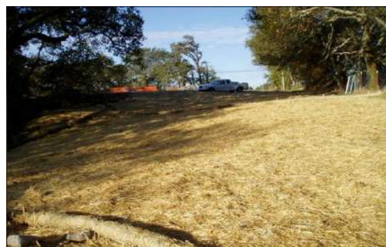
Figure 1-14. Straw mulch covering bare soil to prevent erosion.
