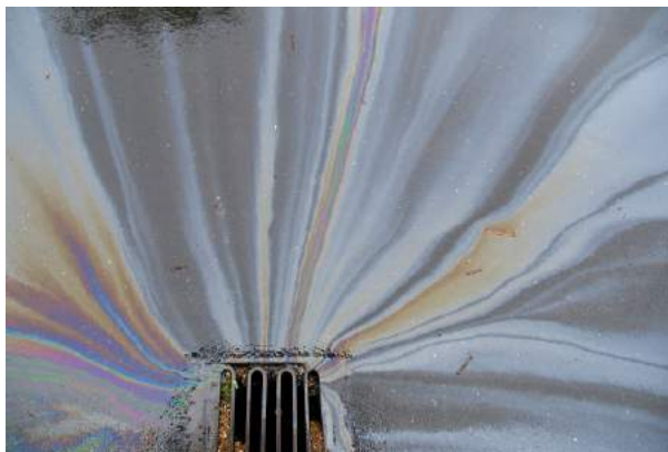
Oil needs to be applied properly so that it does not run off during a rain storm.
